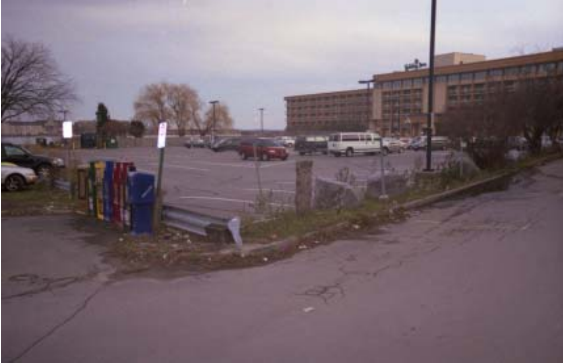
Photo 1: The Accessible Route is currently blocked at the North end of the Holiday Inn Lot
