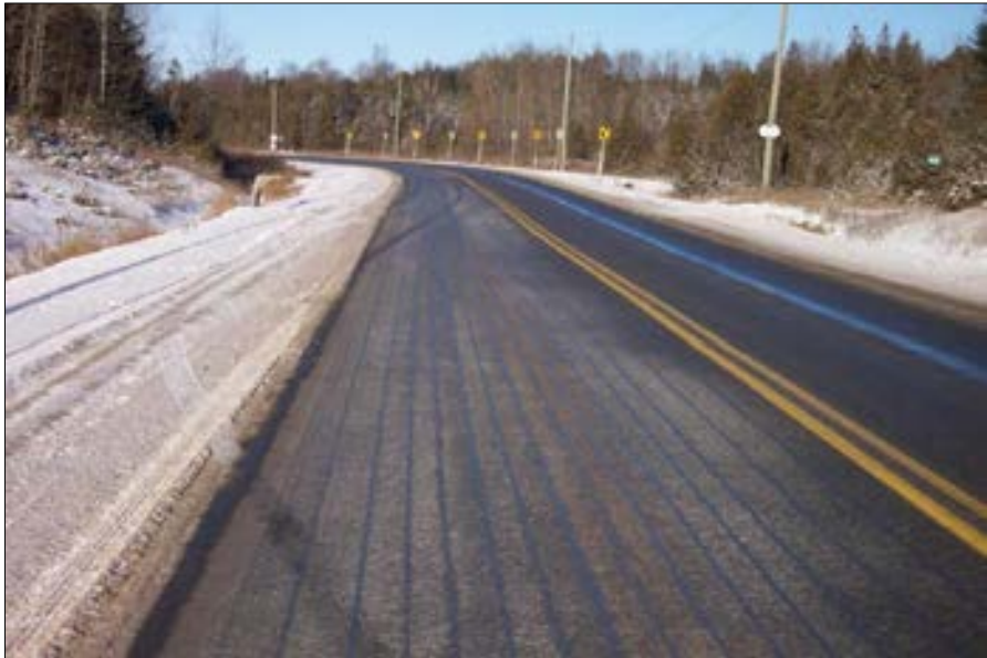
DLA / Anti-icing Application 'Before an Expected Event'
