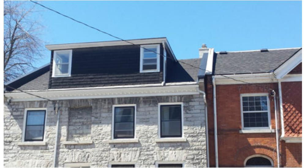
Figure 2: Existing asphalt shingles on shed dormer
