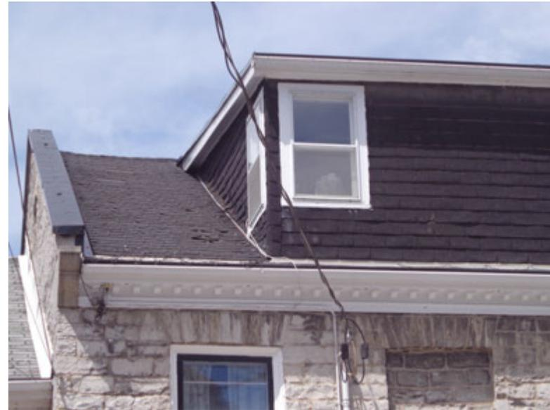
Figure 4: Focus on shed dormer and gable, showing existing condition
