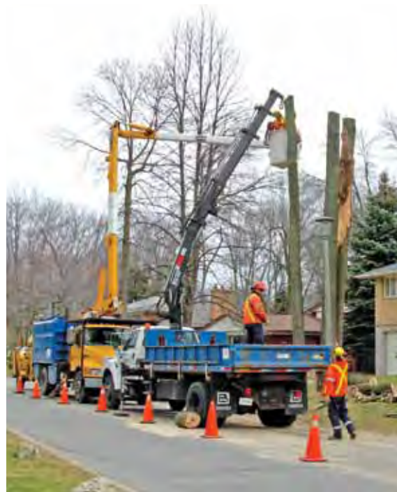
Aerial device and crane
