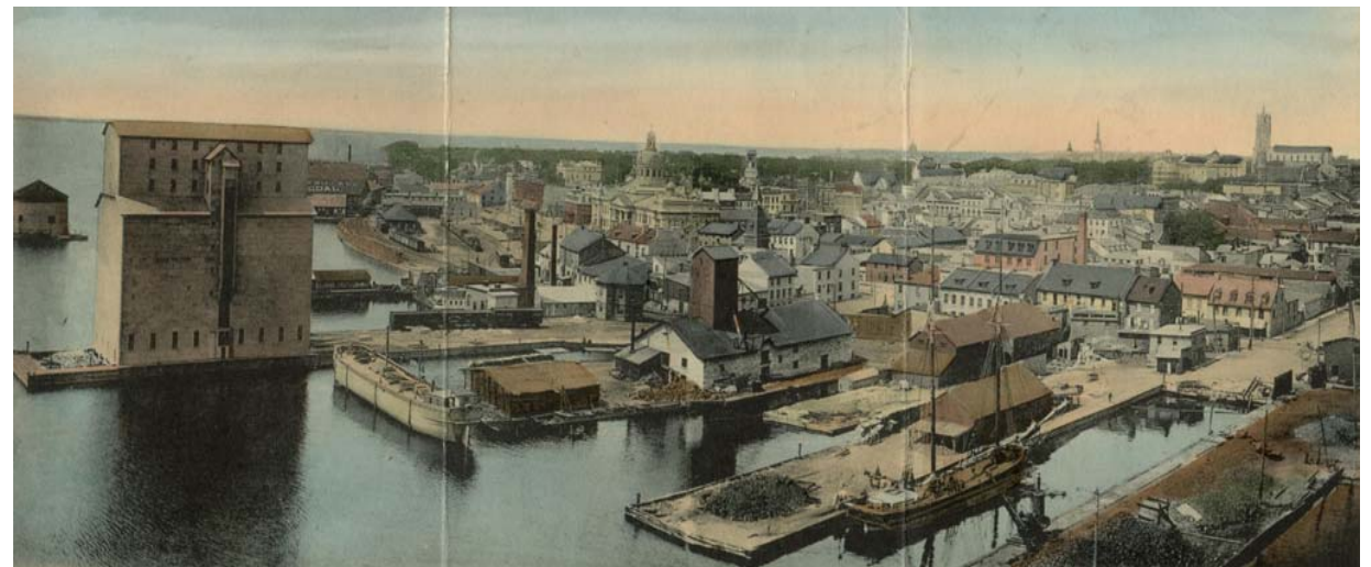
The waterfront quays in the existing Ferry terminal vicinity - from the collections of John Grenville and William Barrow
