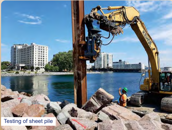
Pile testing in basin
